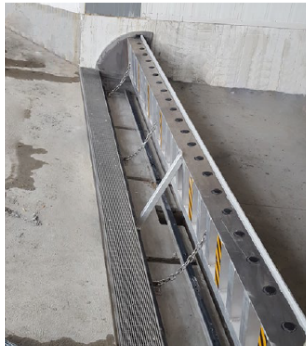
Figure 83. A self-actuating tilting flood barrier protects the entrance to a basement.
